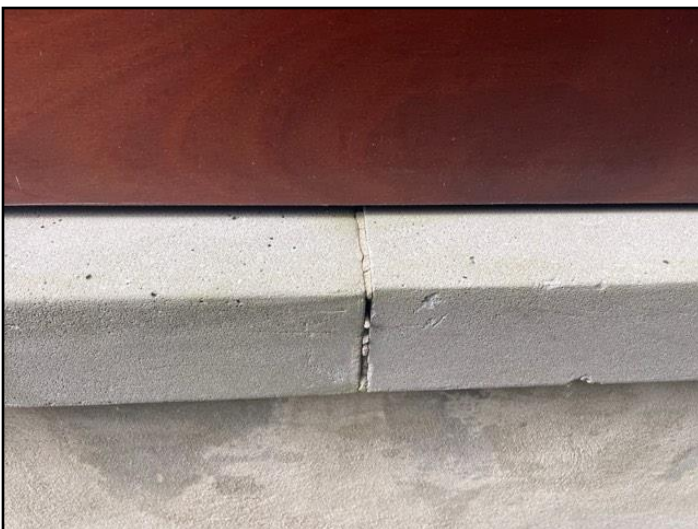
1. Mortar deterioration
