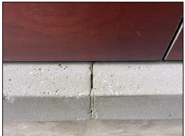
2. Mortar deterioration
